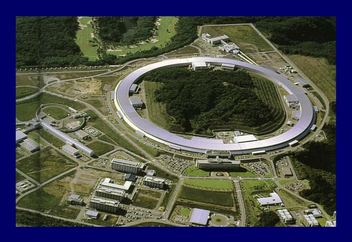
8 GeV electron ring for synchrotron radiation and LEPS GeV gamma rays for nuclear particle physics
